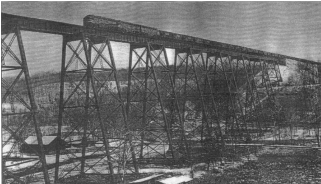
Tinkers Creek Trestle in the Cuyahoga River valley. A westbound train of N&W and C&O hoppers crosses in March 1957. Photo by H.H. Harwood, Jr.
