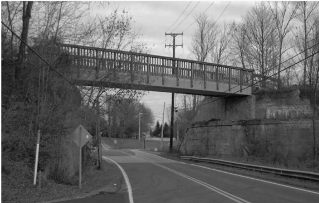
Bike trail crosses over Barlow Road in Hudson. New bridge built on the old railroad abutments. Photo by Gene Stebbins
